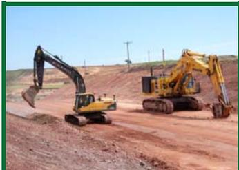
The Hemerdon project has seen an investment of £15M in a brand new Caterpillar equipment fleet, at the core of which are three 110t excavators and twelve 65t rigid dump trucks. Equipment is being operated by a locally recruited workforce, as part of the company's drive to provide employment opportunities in an area with a rich surface mining heritage.
