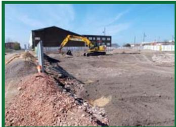
Blackwell was appointed to remediate the site, which was contaminated by a number of known substances including hydrocarbons, heavy metals, metalloids and asbestos. The company also carried out bulk excavation operations and ground shaping earthworks to enable the construction of the required development platforms and landscaped areas.
